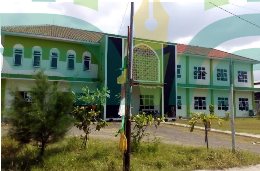
Gedung SMP IT Usamah Boarding School muka depan di pagi hari
